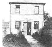
Lombard Street Chapel (Lichfield Methodist Church)
