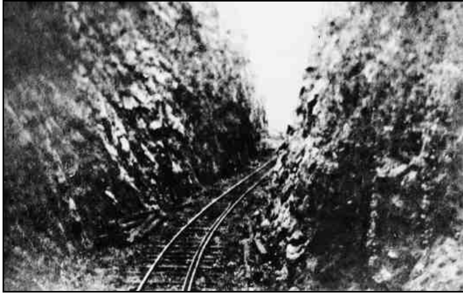
KONYU CUTTING (HELLFIRE PASS) TAKEN SHORTLY AFTER THE END OF THE WAR AND BEFORE THE RAIL LINE WAS REMOVED. THE POWs HAD TO CREATE A RAVINE THROUGH THE ROCKS TO ALLOW THE TRAIN LINE TO PASS THROUGH.
